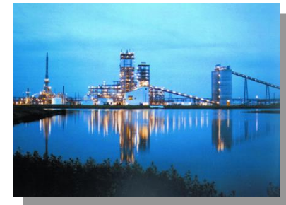
IGCC Power Plant
