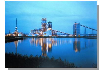
IGCC Power Plant
