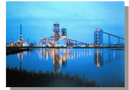
IGCC Power Plant
