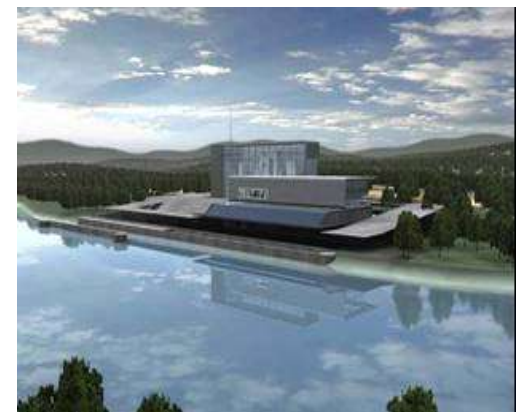
FutureGen Power Plant
