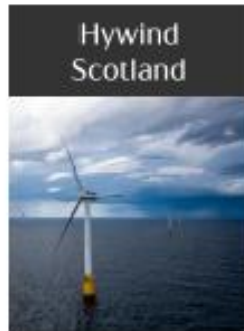
In operation Offshore floating wind
