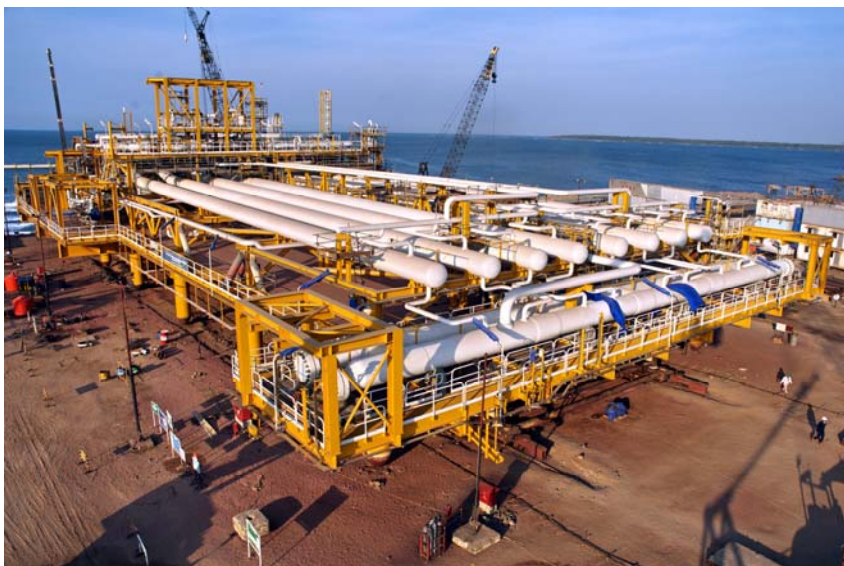
Total Indonesia slug catchers: 3200t, 14 legs ECCE – September 2011
